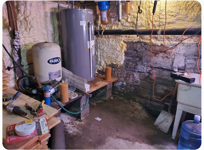
General photo of the water tank; partial insulation of exterior walls
