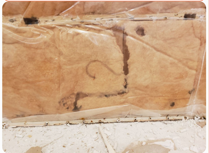
Remediation Project: August 12, 2022; An evidence of mice droppings was found
