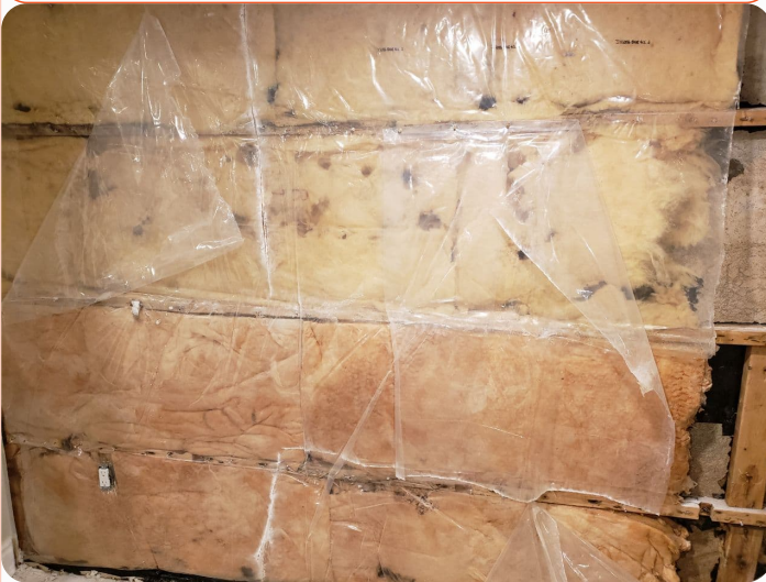
Remediation Project: August 12, 2022; Containment setup
