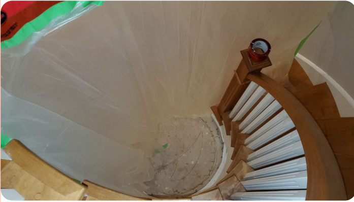
Remediation Project: August 12, 2022; Containment setup
