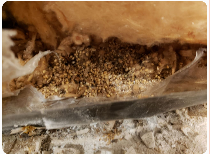
Remediation Project: August 12, 2022; An evidence of mice droppings was found
